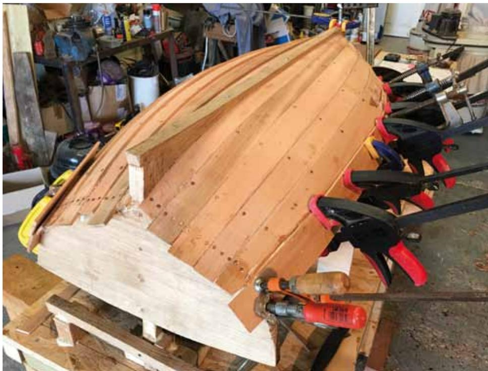
were needed and my experience is that a number always break when being fitted. So I prepared 20. But when the job was done not one timber had broken; if I had only made 14, I would have broken the lot no doubt.
